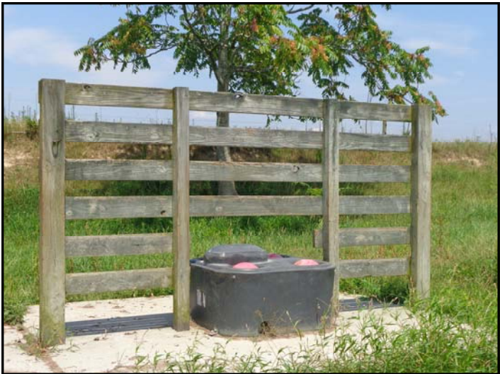
Waterer fed by gravity from holding tank from solar panel.
