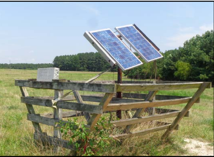
Solar panel for pumping water to holding tanks.
