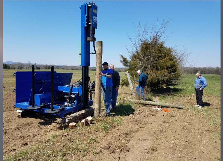
Line post can be placed on 10' to 25' centers depending on layout and terrain covered.
