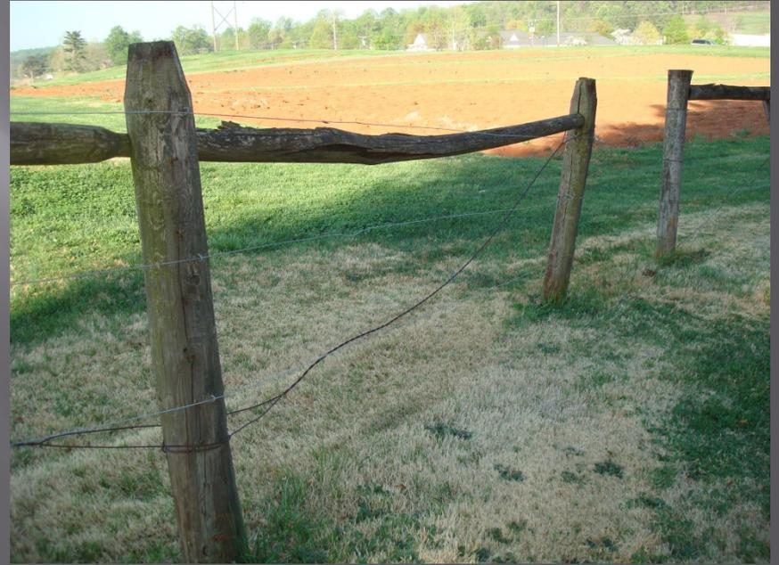
H braces are the foundation of any fence and are critical to life of your system.
